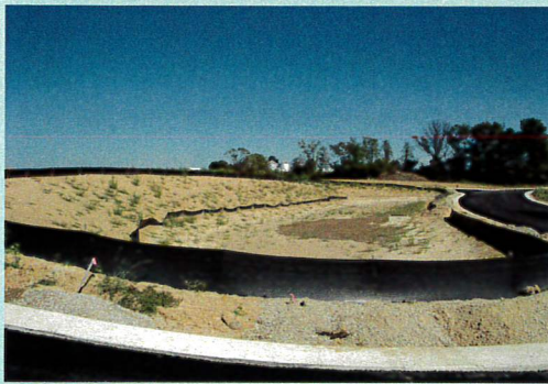
A rain garden during construction in Wood River, Illinois (William Freeman)
