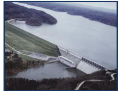
Dams vary in size and shape, the amount of water they impound, and their assigned hazard classification.
