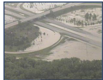
When large highways close due to flooding, traffic is detoured causing inconvenience and economic loss.
